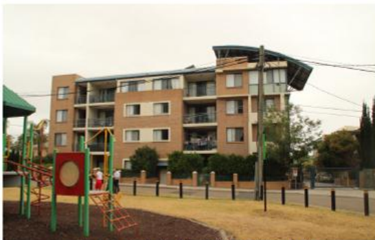
Playground and residential flat building behind on Marsden Street
