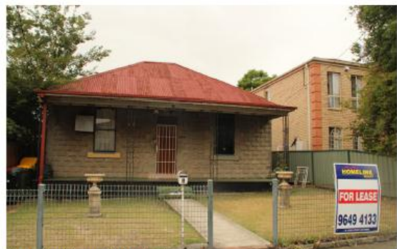
Single dwelling at 1 Marsden Street
